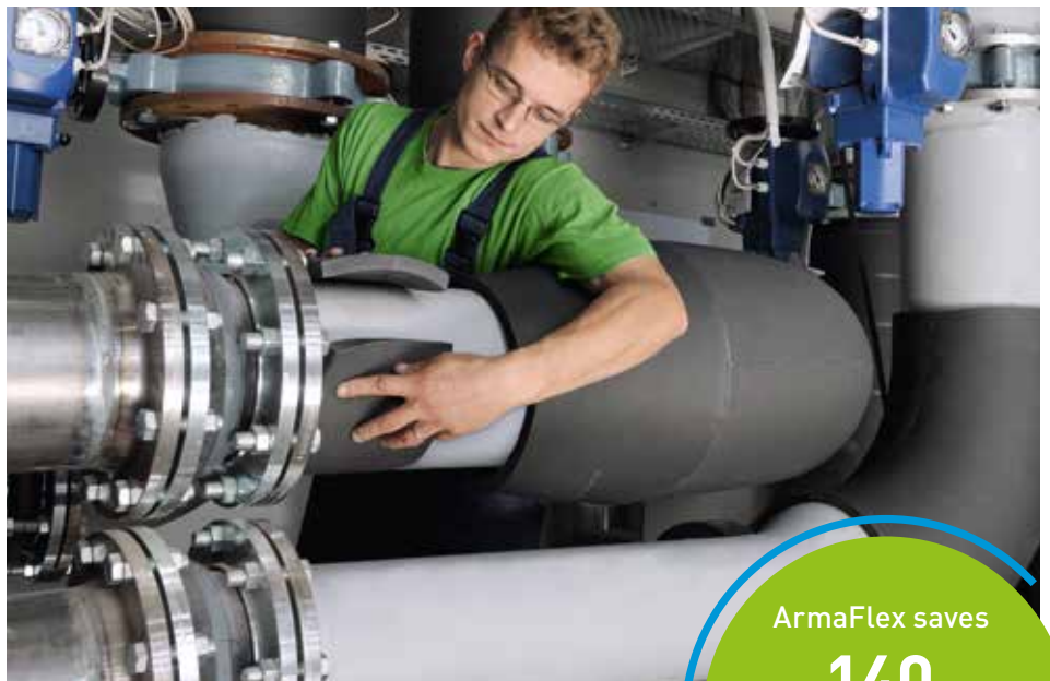
While accounting for an average of just 1 percent of the total costs of the technical equipment, insulation materials ensure higher performance, a longer service life and higher efficiency
