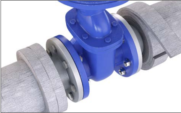
Figure 58: Preparation for valve cover.
