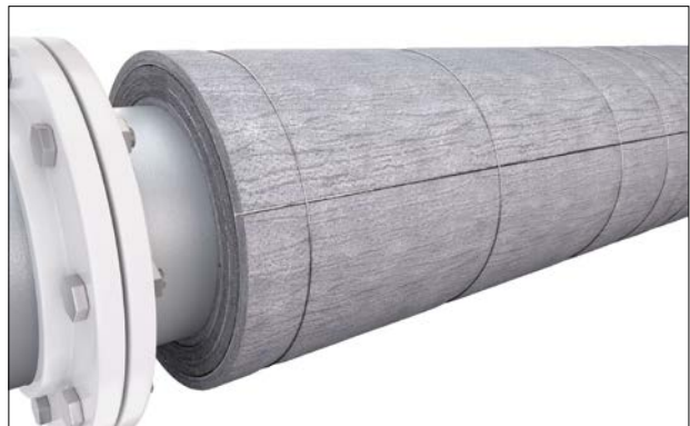
Figure 24: Positioning of final layer.
