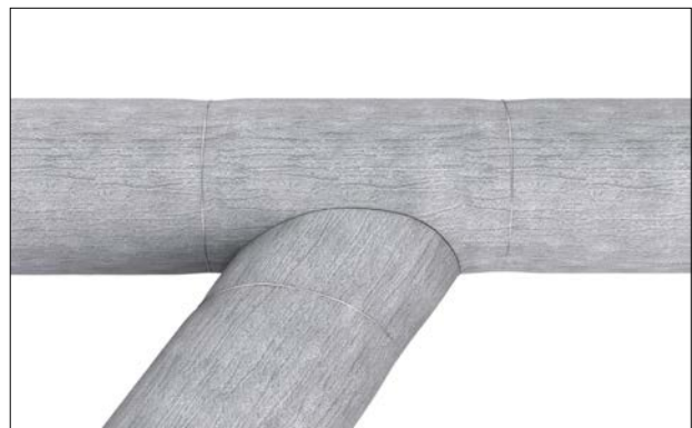
Figure 55: Completed tee cover.
