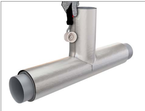
Figure 76: Securing joints with roller
