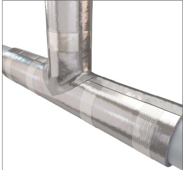
Figure 29: Securing vapour barrier tape
