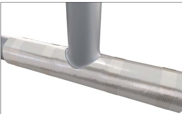
Figure 23: Securing insulation layer with filament tape
