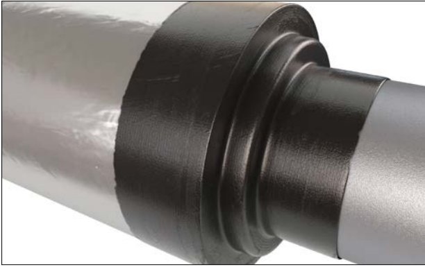
Figure 13: Application of vapour stop at insulation termination
