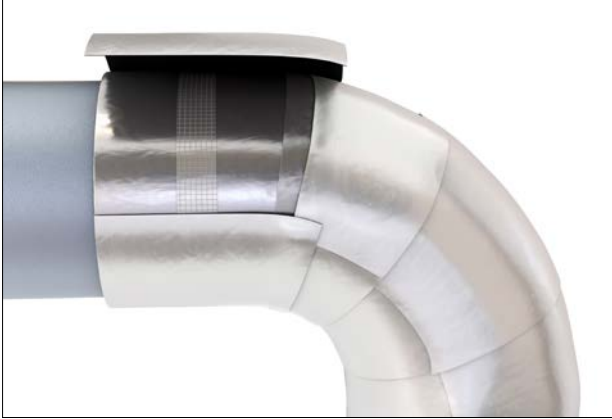
Figure 68: Applying last segment of primary vapour barrier
