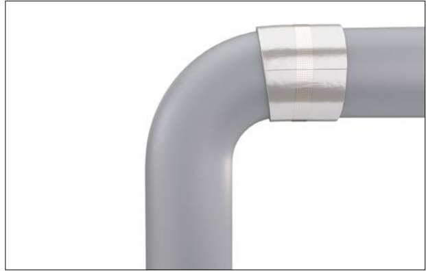
Figure 17: Application of starter segment
